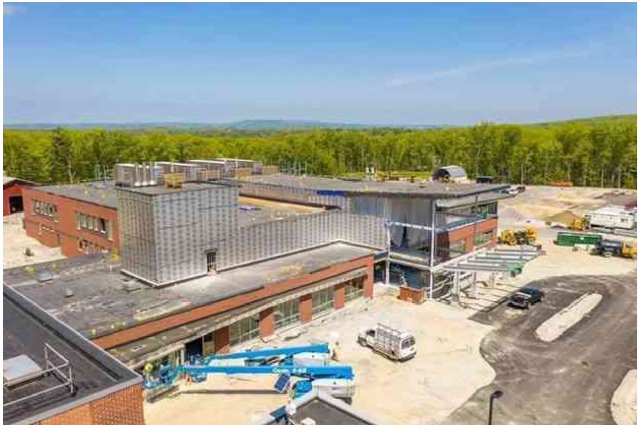
New Dartmouth-Hitchcock Manchester campus construction is on target for February occupancy.
